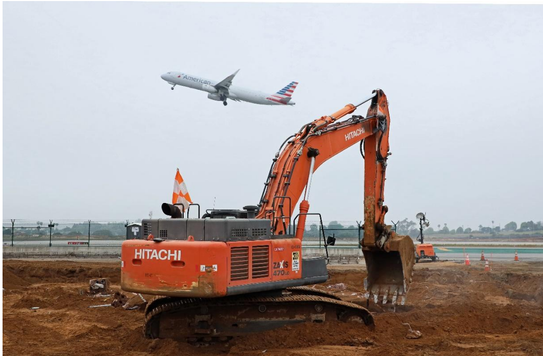
Taxiway Delta Extension at Los Angeles International Airport (2023) – © Colas
